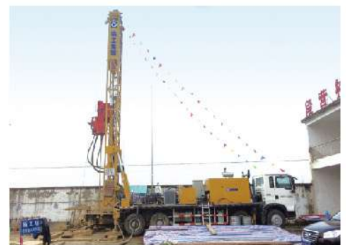
XSC5/260水井钻机亳州水文监测井施工 XSC5/260 Water Well Drilling Rig in Hydrological Monitoring Well Construction in Bozhou
