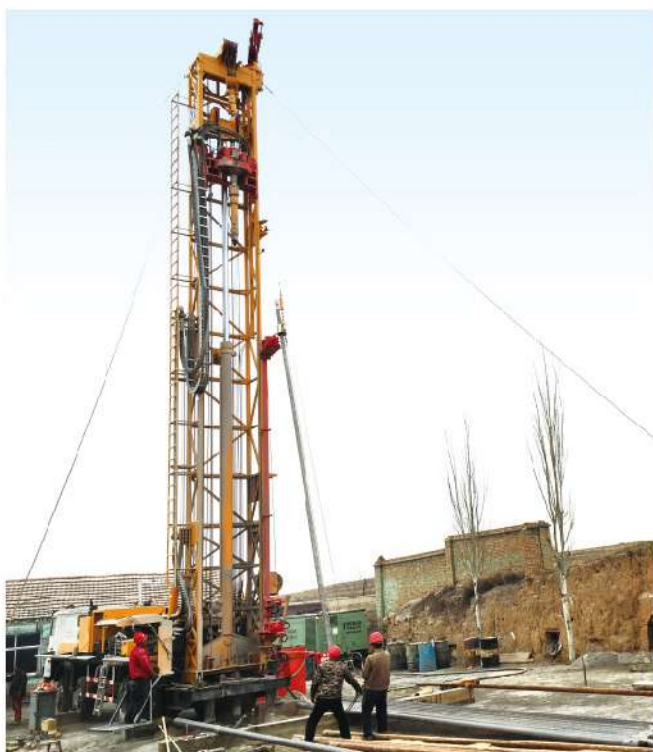
XSC8/400深井钻机山西水井施工 XSC8/400 Deep Well Drilling Rig in Water Well Construction in Shanxi
