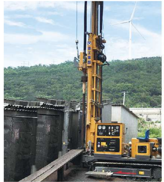
XSL4/200水井钻机福建饮水井施工 XSL4/200 Water Well Drilling Rig in Water Well Construction in Fujian
