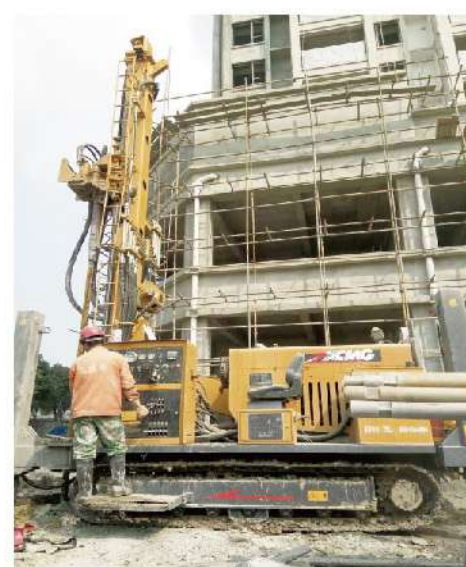
XSL5/260水井钻机湖北地热井施工 XSL5/260 Water Well Drilling Rig in Geothermal Well Construction in Hubei
