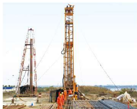
XSC8/400深井钻机盐城水文监测井施工 XSC8/400 Deep Well Drilling Rig in Hydrological Monitoring Well Construction in Yancheng
