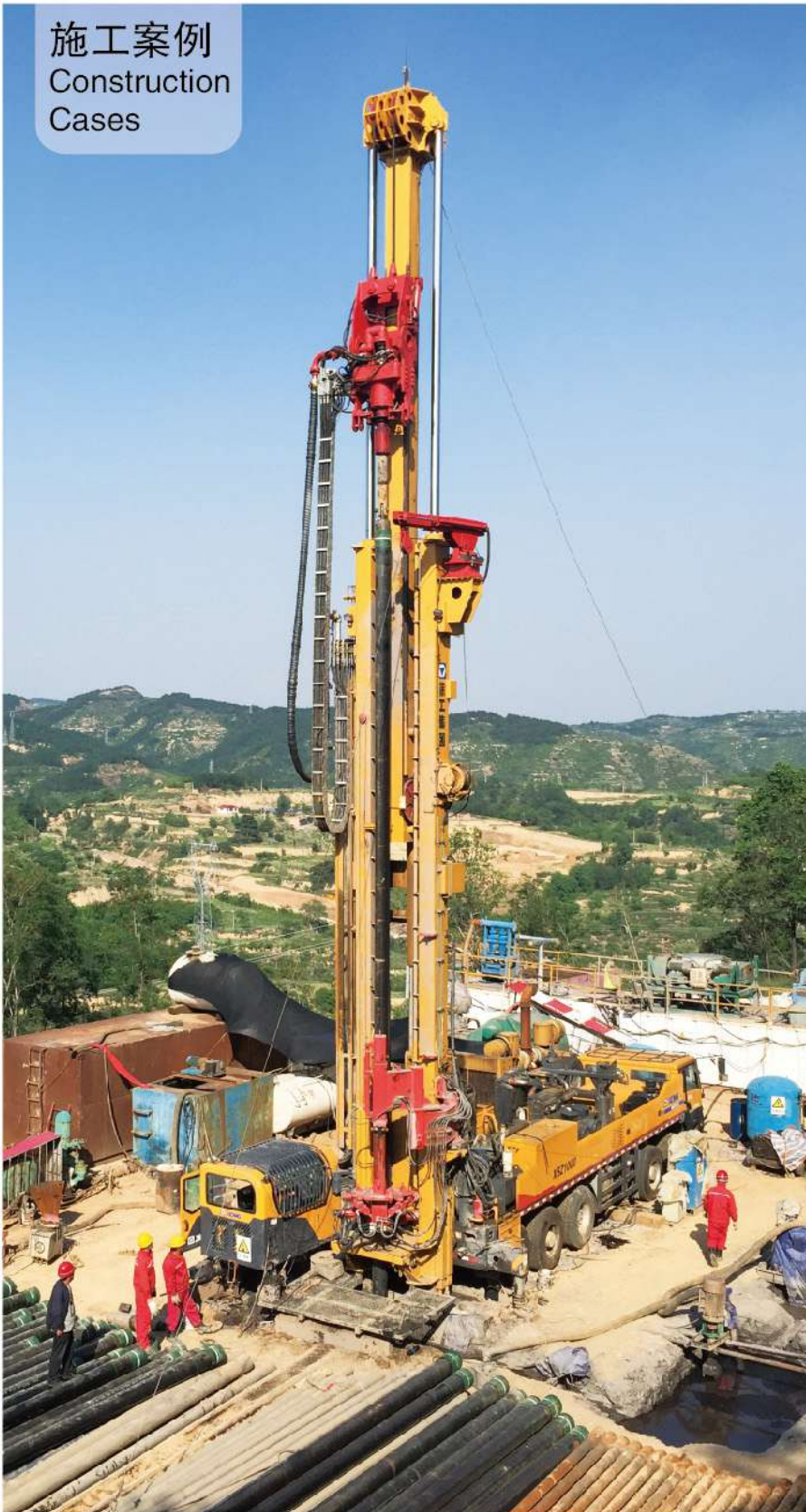
XSC20/1000深井钻机山西煤层气井施工 XSC20/1000 Deep Well Drilling Rig in CBM Well Construction in Shanxi
