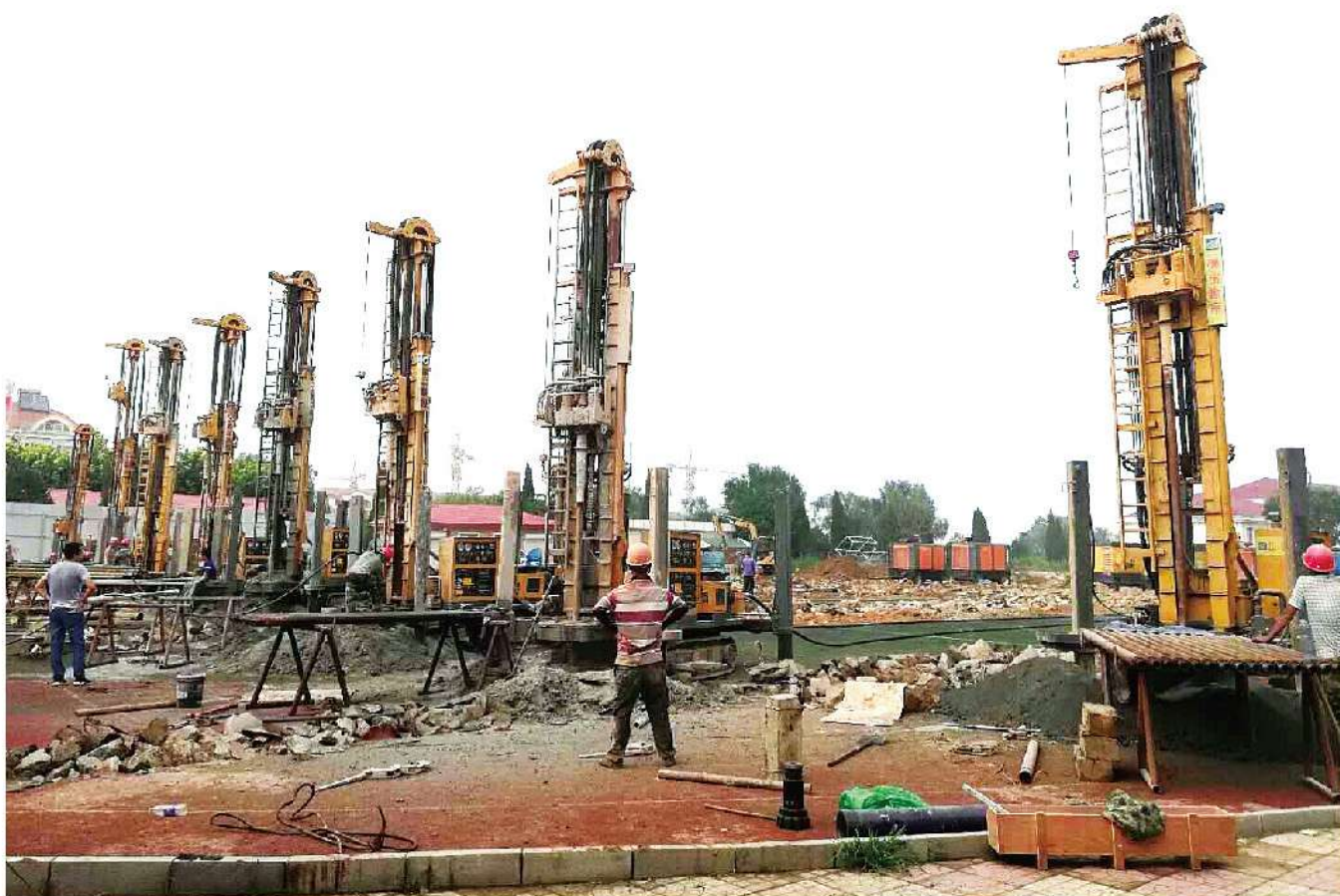
XSL4/200水井钻机北戴河地热井施工 XSL4/200 Water Well Drilling Rig in Geothermal Well Construction in Beidaihe
