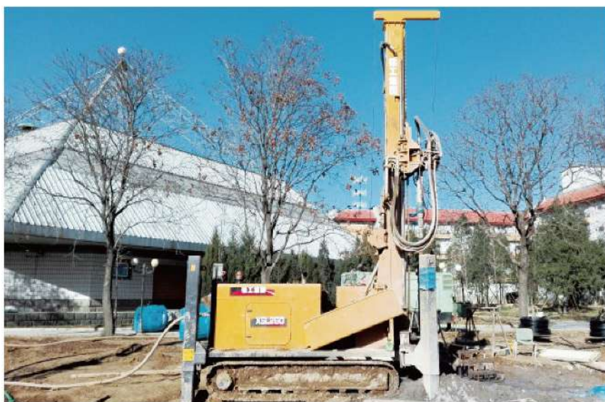
XSL5/260水井钻机北京地热井施工 XSL5/260 Water Well Drilling Rig in Geothermal Well Construction in Beijing
