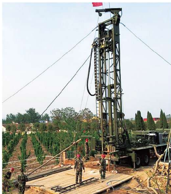
XSC8/400深井钻机河南水井施工 XSC8/400 Deep Well Drilling Rig in Water Well Construction in Henan
