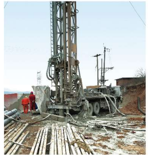
XSC8/400深井钻机山西煤层气井施工 XSC8/400 Deep Well Drilling Rig in CBM Well Construction in Shanxi
